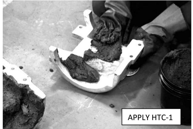
4. **Install ControHeat** – Place HTC-1 coated ControHeat jacket pieces back on the component and use the fasteners supplied to draw the pieces together. Extra torque may be required to get the HTC-1 to conform to the clearance between the ControHeat and component. HTC-1 should squeeze out of jacket, if no excess HTC-1 is present, not enough compound was applied during step 3.
