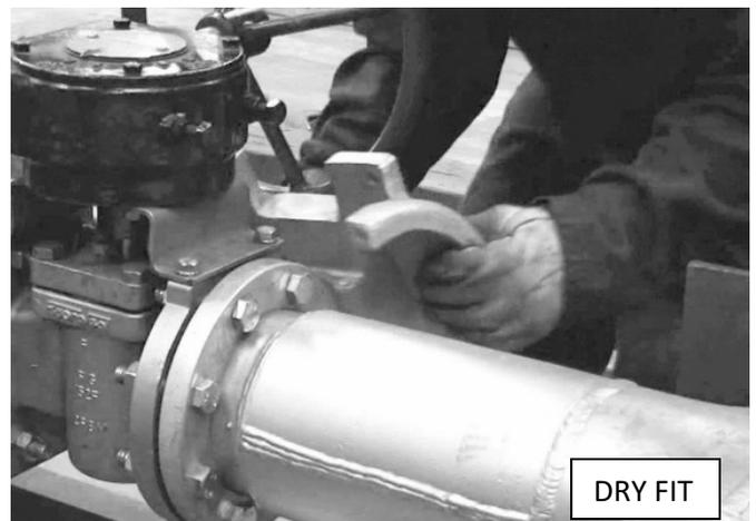
3. **Apply HTC-1** - Remove dry fitted jacket pieces from the component and apply HTC-1 to interior of the ControHeat jacket pieces using gloves or trowel.
