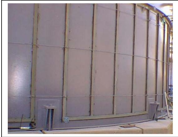
Picture 1 – ControTrace External Tank Jacket
